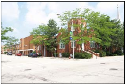
PROPERTY TO NORTH 3 302 N DUNTON AVE
