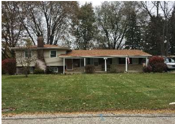
Property Across 1310 W. Hawthorne
