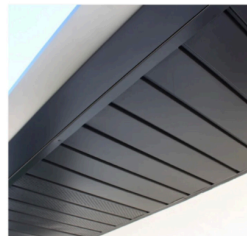
Black fascia and gutters
