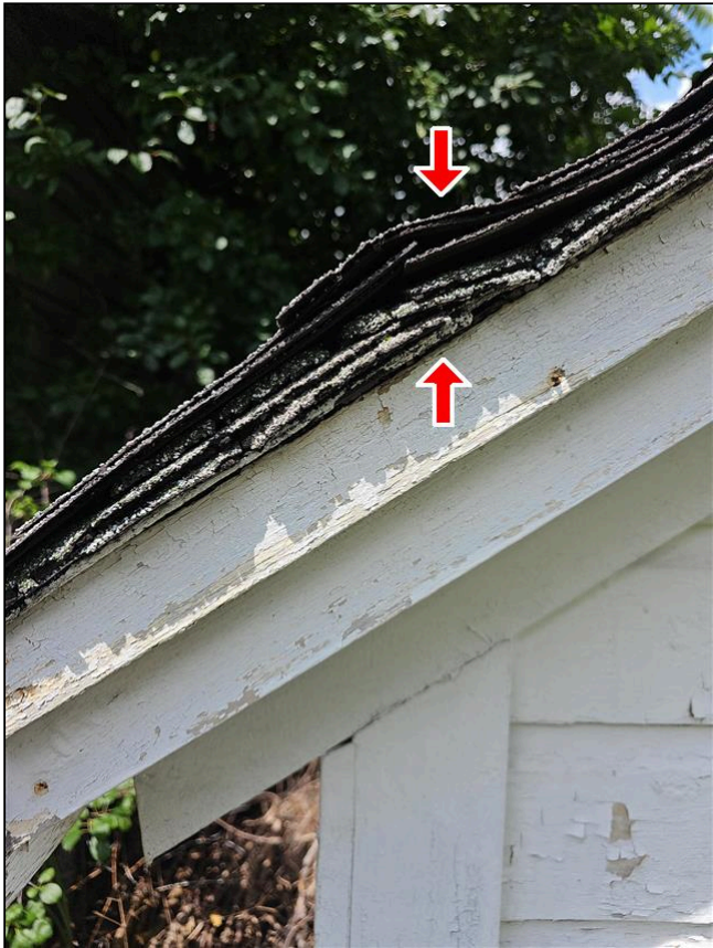
3.0 Item 7(Picture) Roofing
