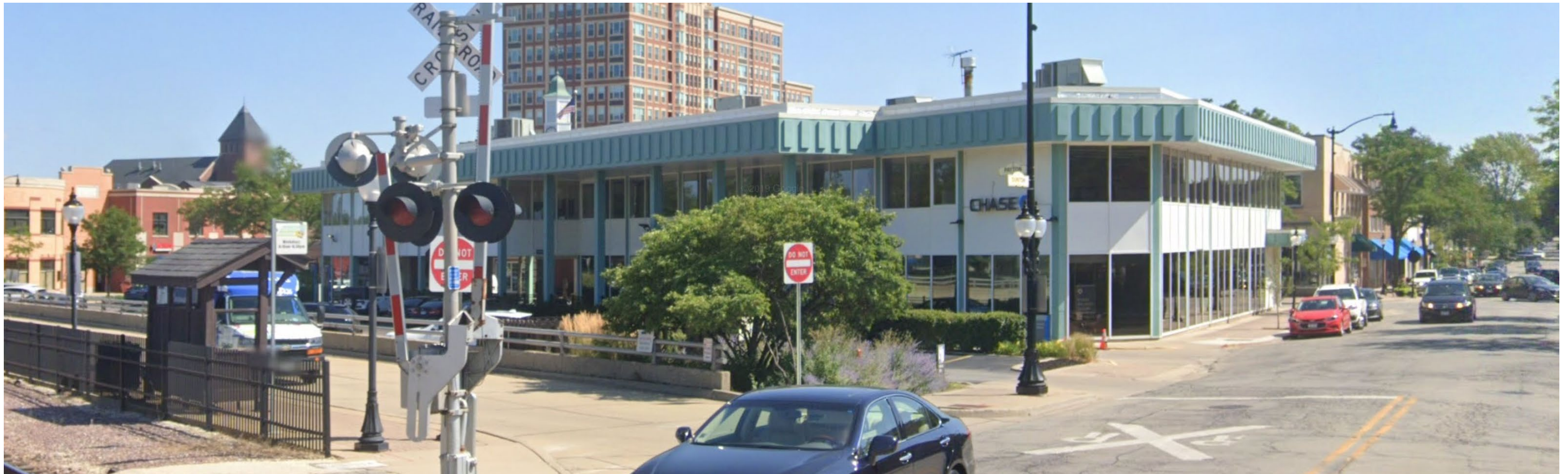
VIEW OF ROOFTOP MECHANICAL EQUIPMENT FROM DUNTUN AVENUE
