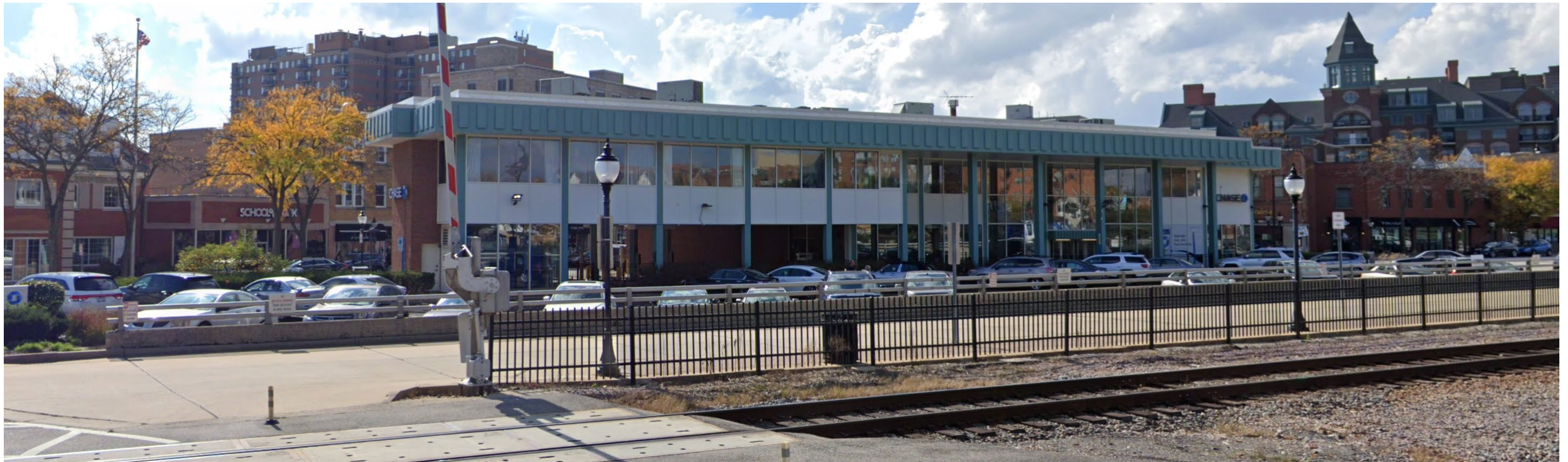
VIEW OF ROOFTOP MECHANICAL EQUIPMENT FROM EVERGREEN AVENUE
