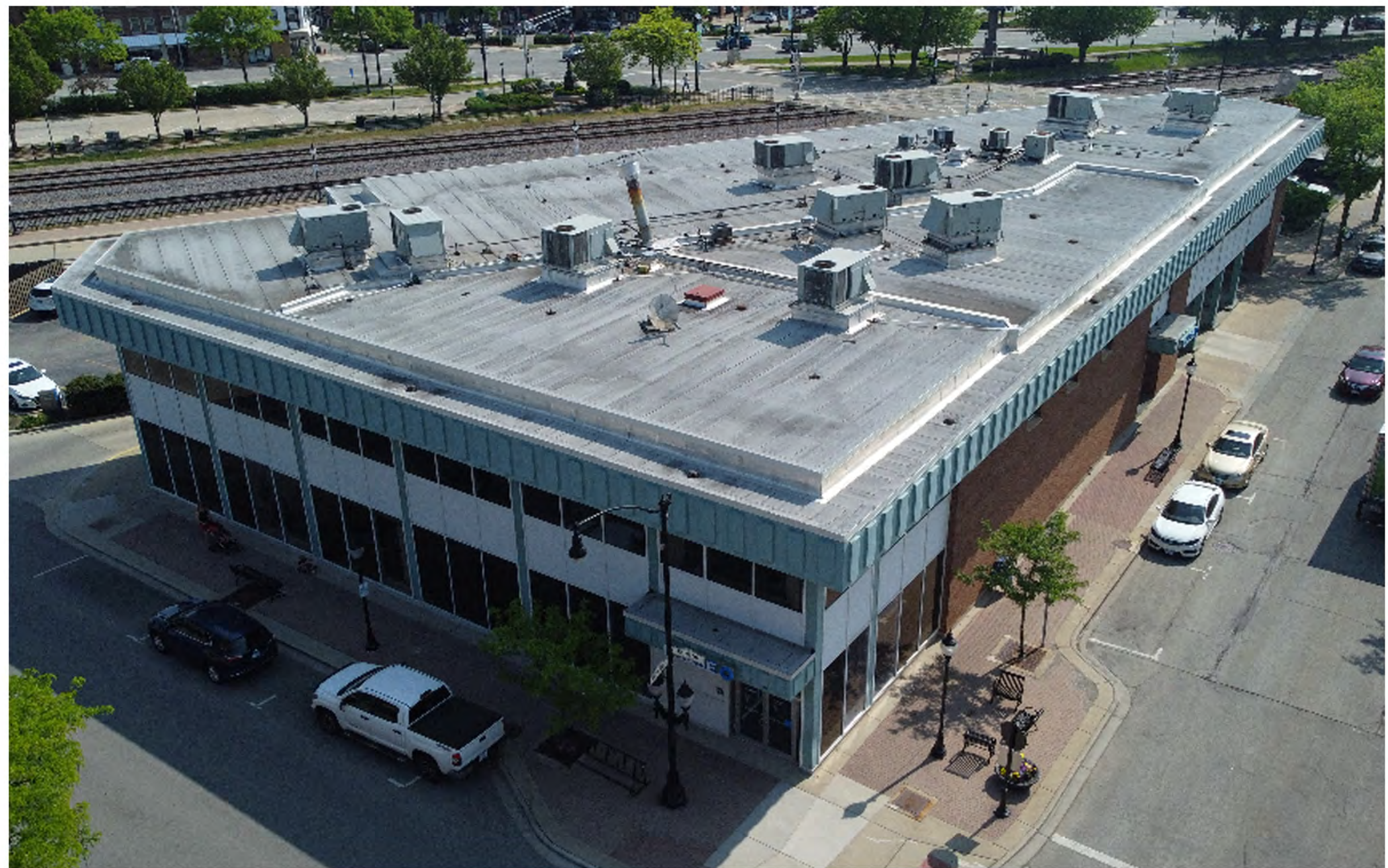
EXISTING ROOF MECHANICAL UNITS
