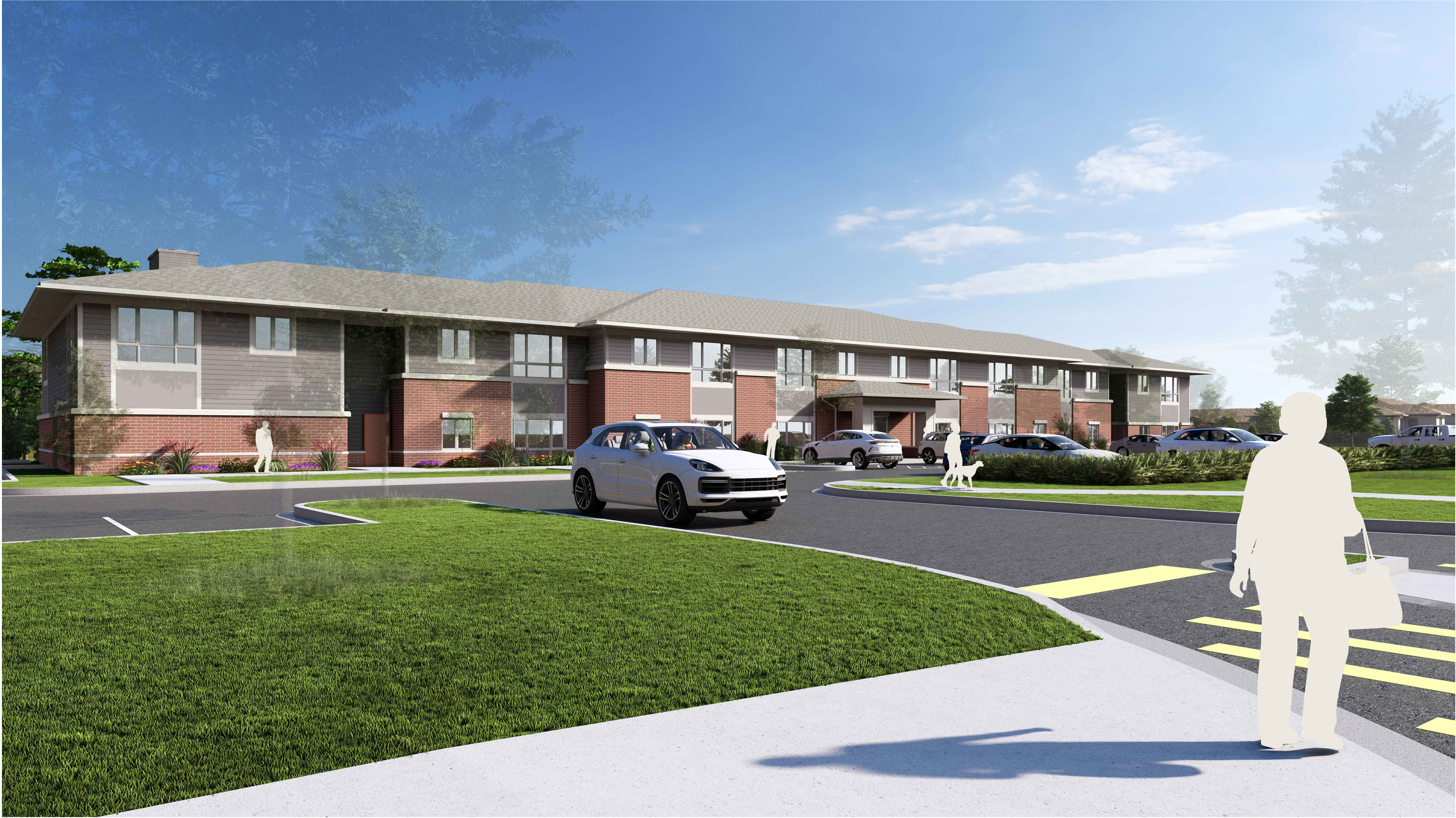
1 NORTH WEST VIEW
