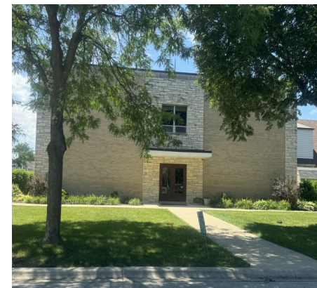
PROPERTY ACROSS 3 431 PINE AVENUE
