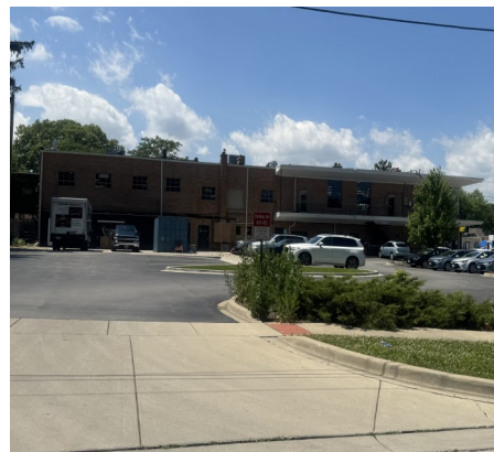
PROPERTY ACROSS 2 413 PINE AVENUE
