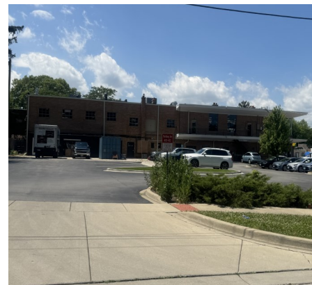
PROPERTY ACROSS 2 413 PINE AVENUE
