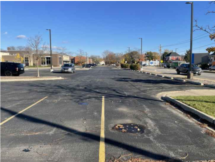
#2-VIEW EAST FROM SITE
