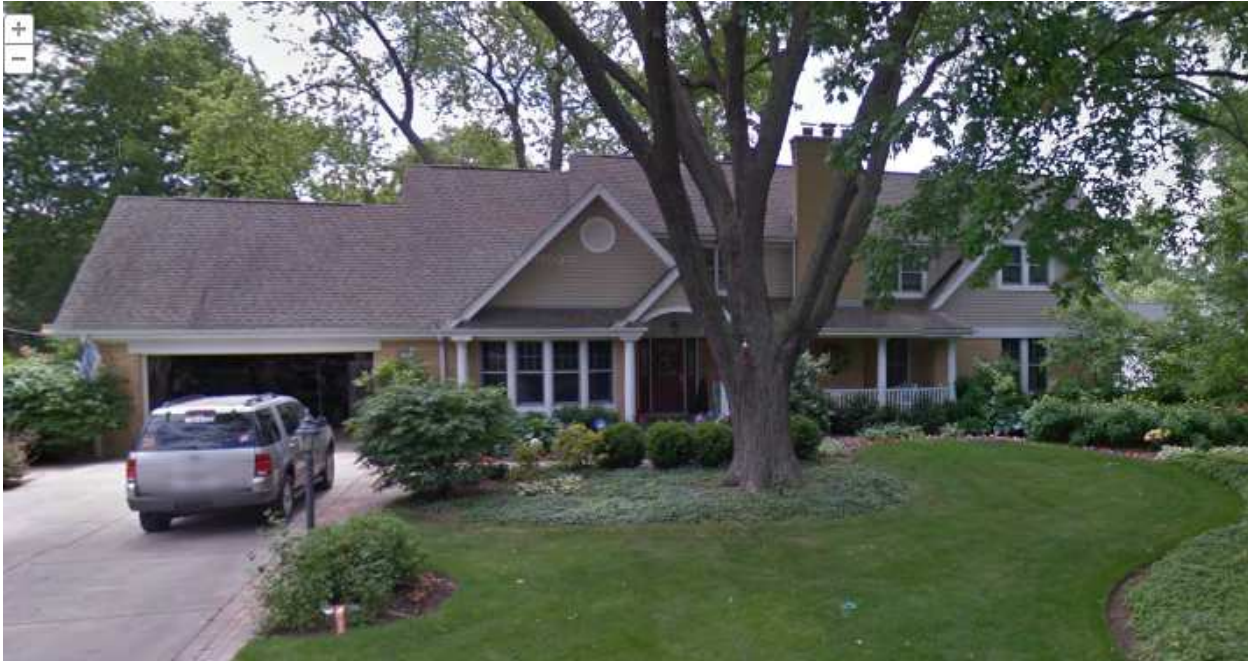
Image 2, 1303 W. Watling Street. This home is a wonderful example of a second story addition to an existing single story house. The gable roof forms and front porch keep the scale of the expanded home within the context of the neighborhood.
