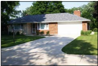
SUBJECT PROPERTY 130 S. FERNANDEZ AVE.
