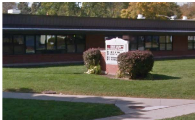
Image 6. Dryden Elementary School
