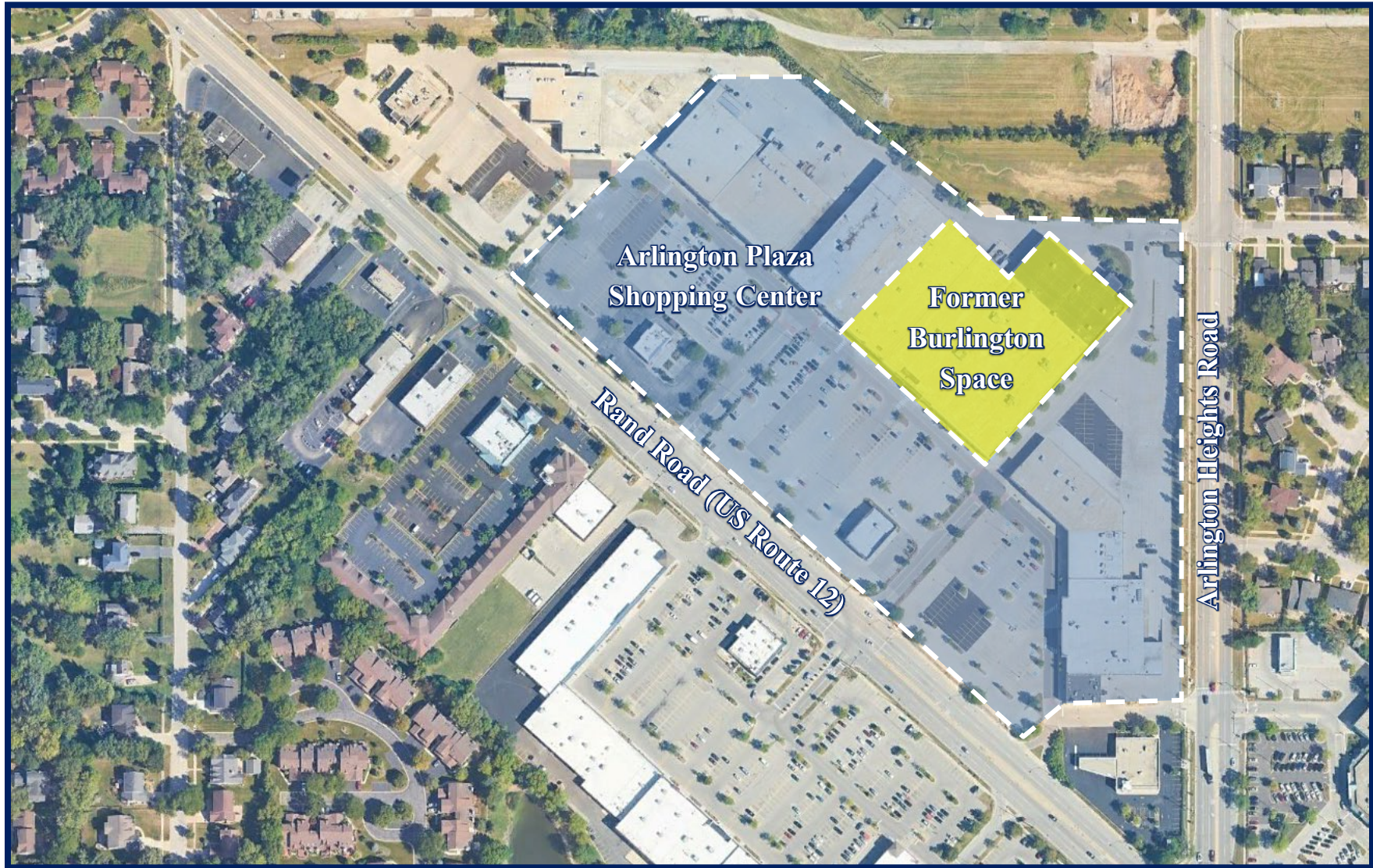
Aerial View of Site
