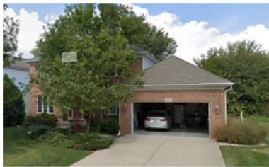
PROPERTY TO LEFT 3 490 E HAVEN ST
