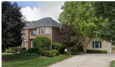
PROPERTY TO LEFT 1 480 E HAVEN ST
