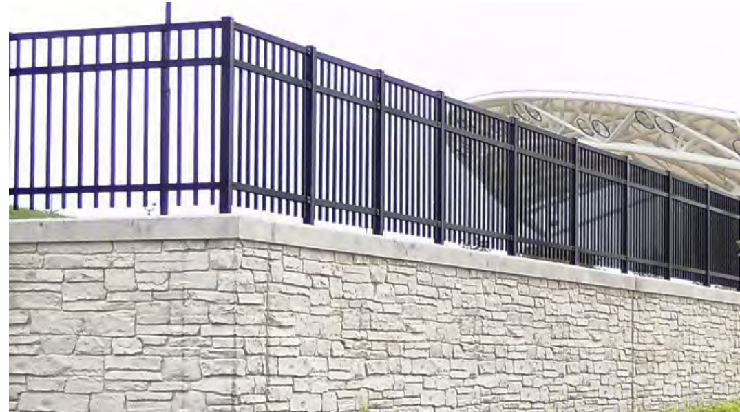
PROPOSE CONCRETE WALL - STONE PATTERN
