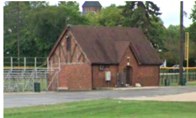
EXISTING STORAGE BUILDING
