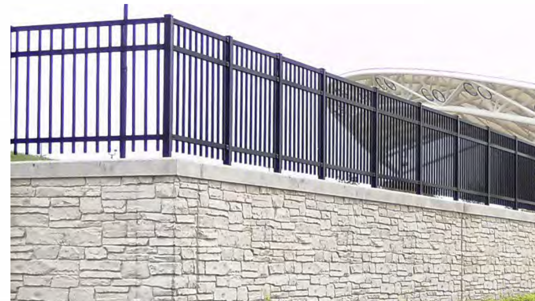
PROPOSE CONCRETE WALL - STONE PATTERN
