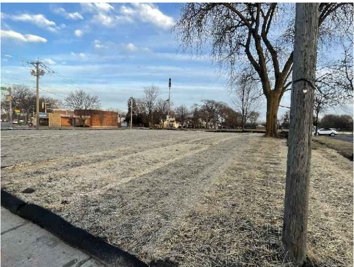
#8-VIEW NW- POST DEMO SITE DEMO COMPLETE LATE FALL '24
