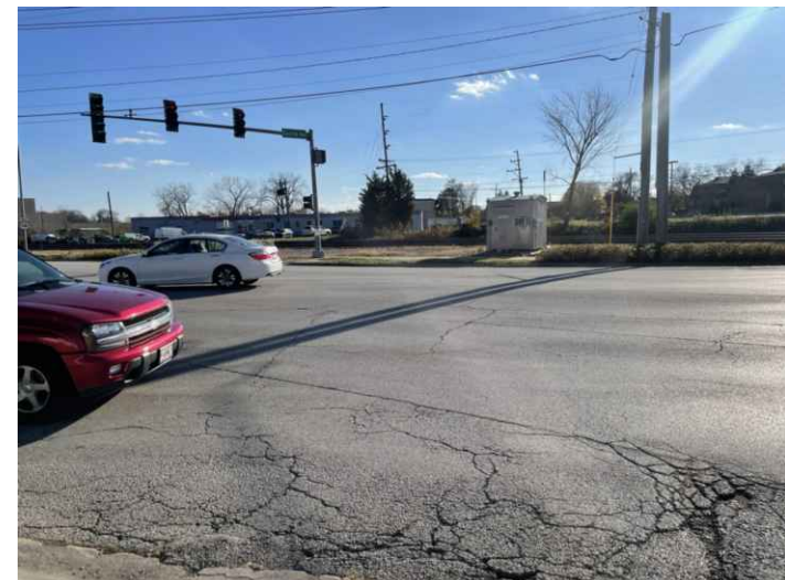
#4-VIEW SOUTHWEST AT SITE
