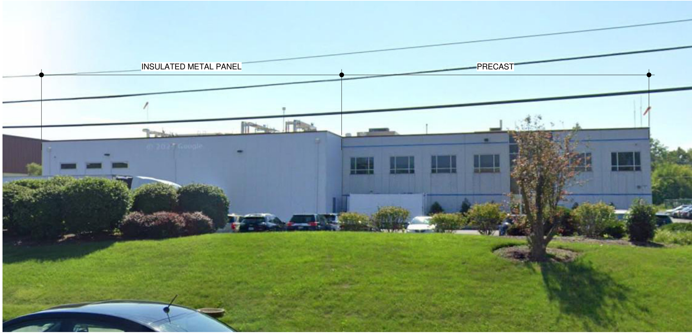
EXISTING TASTY BREADS NORTHBROOK FACILITY
