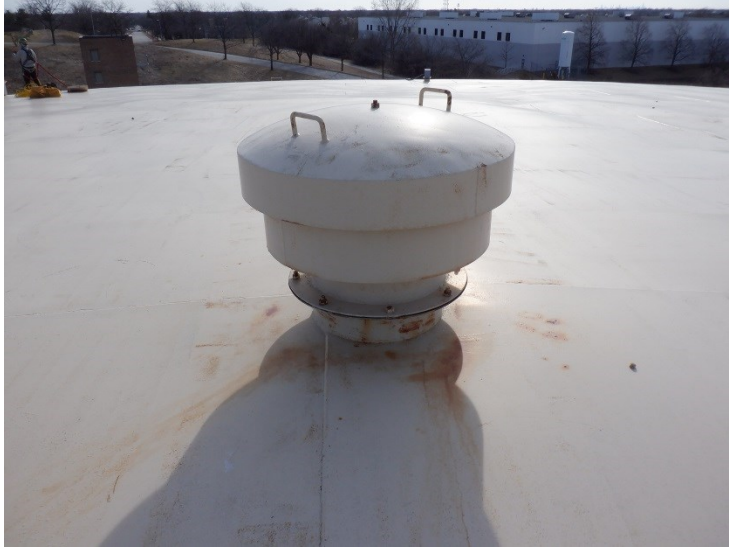
25) The pressure vacuum vent is in fair condition.
