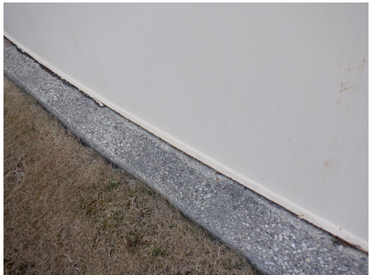
2) The exposed concrete foundation is in good condition overall.
