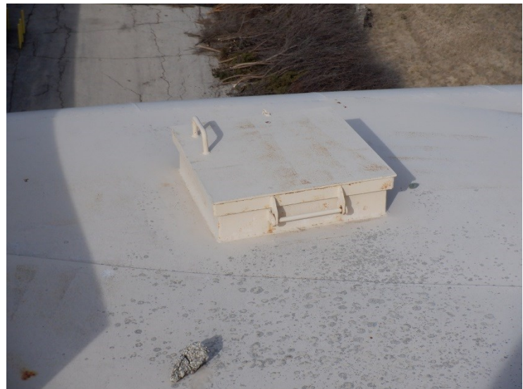
32) The two wet interior roof hatches are in good condition.
