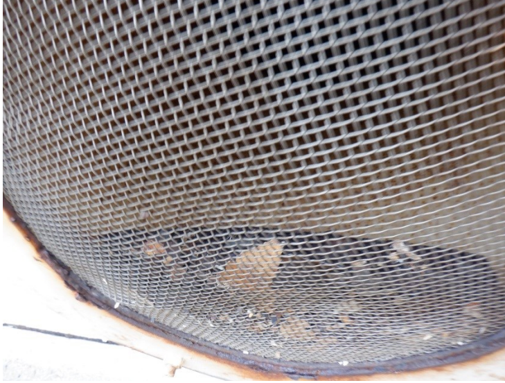
16) The overflow pipe screen is in good condition. The screen is oversized.
