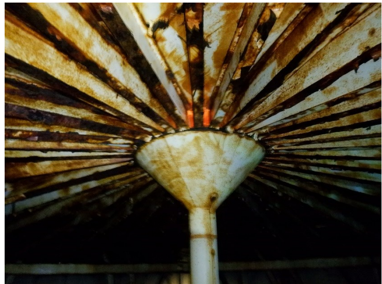
35) The center support column is in good condition but restricts the exchange of air for venting purposes
