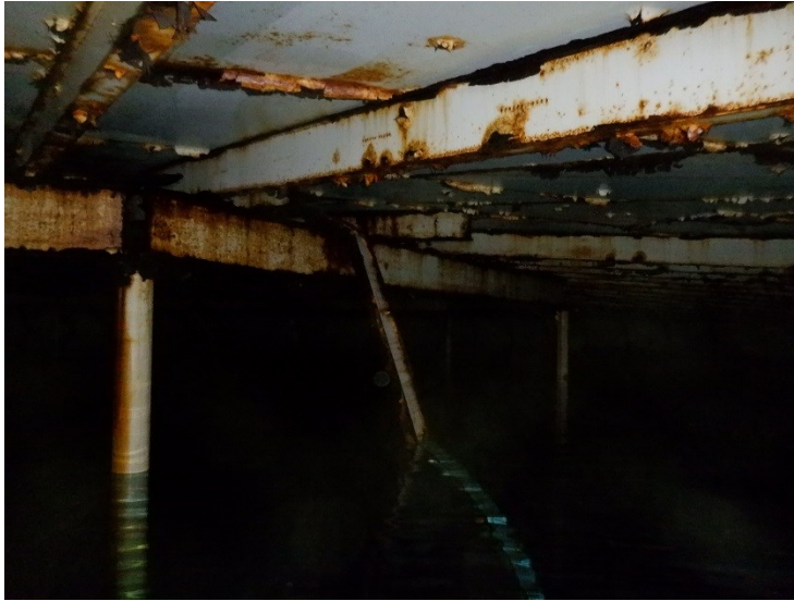
37) There are several beams hanging from the roof.
