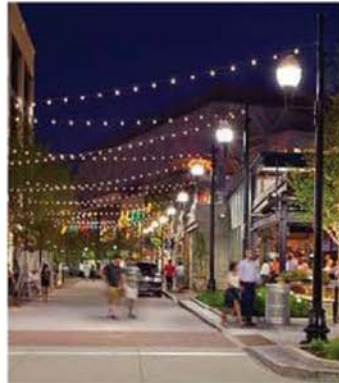
Pedestrian Light with Catenary Lights Sternberg Lighting Custom
