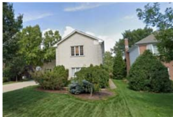
PROPERTY TO LEFT 2 484 E HAVEN ST
