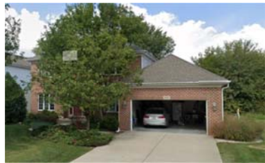
PROPERTY TO LEFT 3 490 E HAVEN ST
