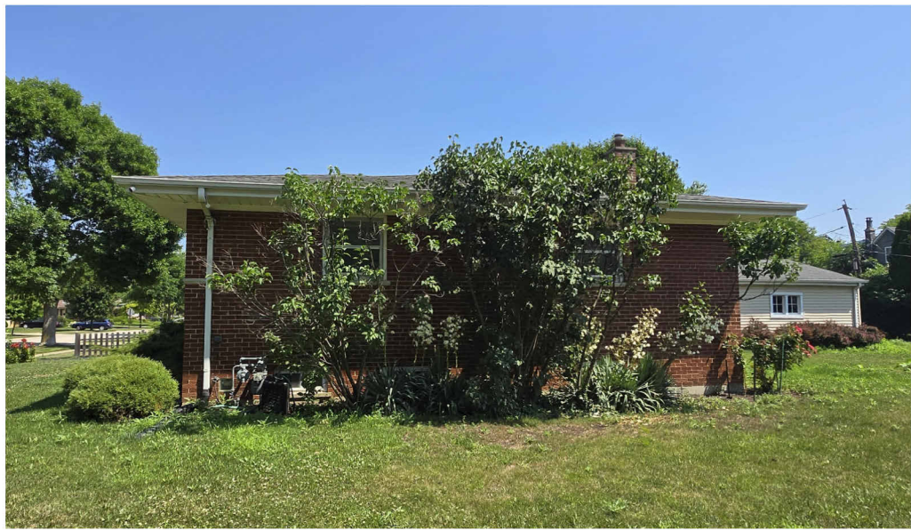
603 N Wilshire Ln Euclid Ave view
