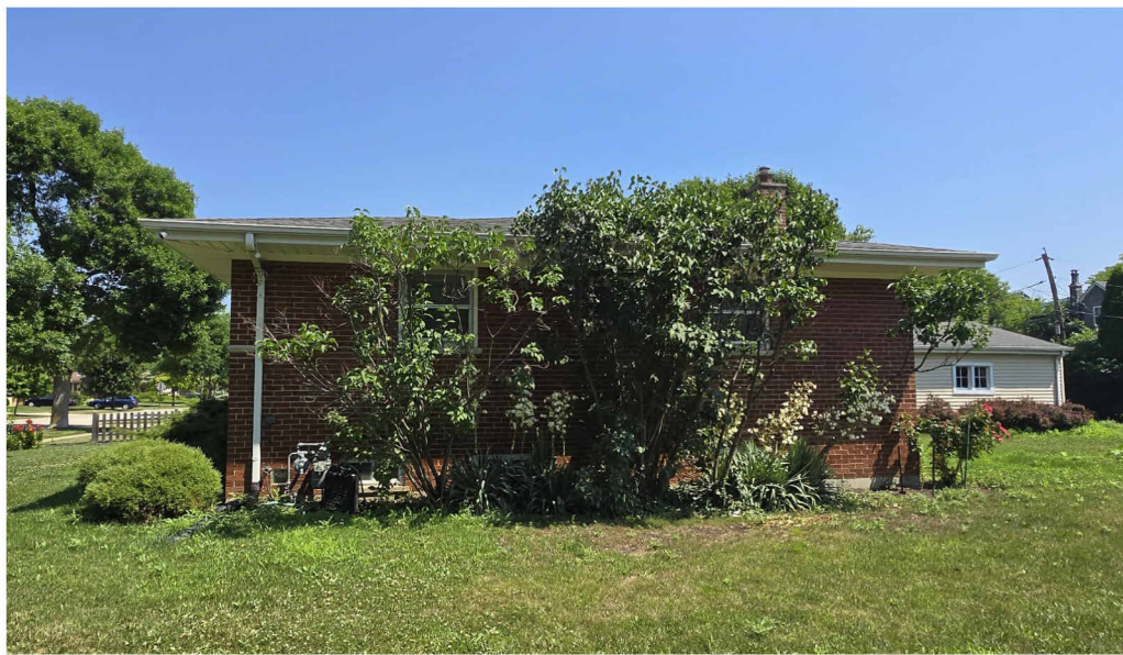
603 N Wilshire Ln Euclid Ave view
