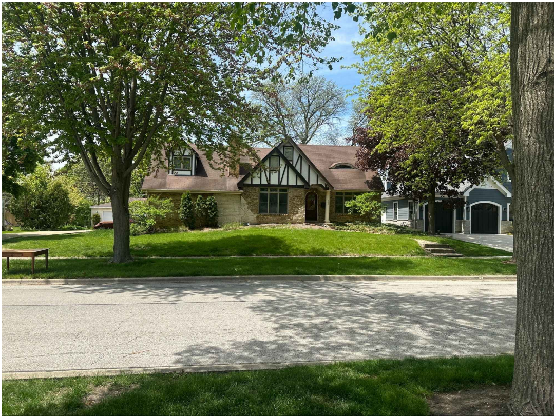
704 S. MITCHELL AVE. SUBJECT PROPERTY
