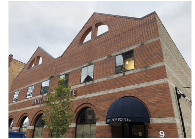
C N. VAIL AVE. PUBLIC SIDEWALK AND PROPERTY'S FRONT FACADE
