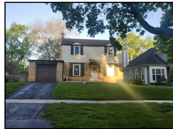
636 SOUTH MITCHELL AVE. PROPERTY TO SOUTH 3
