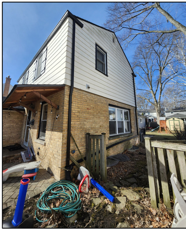
photo of existing - north
