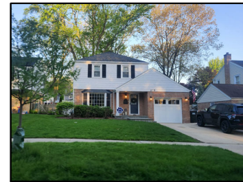
618 SOUTH MITCHELL AVE. PROPERTY TO NORTH 1
