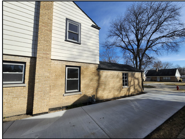
photo of existing - south
