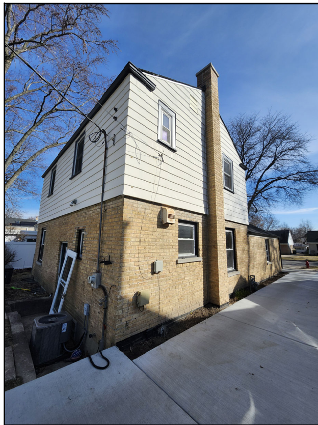
photo of existing - south
