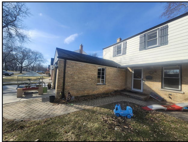
photo of existing - north
