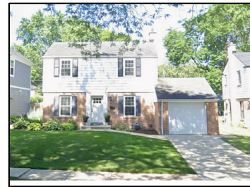
626 SOUTH MITCHELL AVE. PROPERTY TO SOUTH 1
