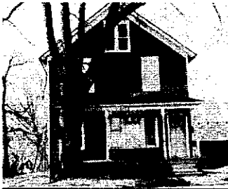
204 S. Arlington Heights Rd. DEMOLISHED
