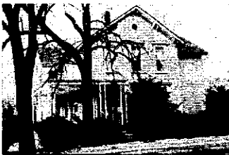
210 S. Arlington Heights Rd. DEMOLISHED
