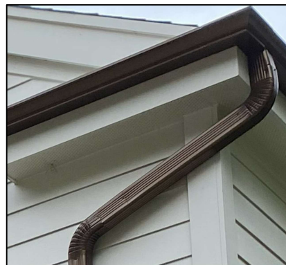
GUTTERS / DOWNSPOUTS: - ALUMINUM, BROWN T.M.E.
