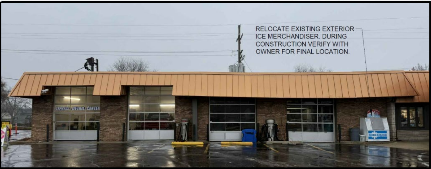
3 BUILDING SOUTHWEST VIEW A2.0 Scale: N.T.S.
