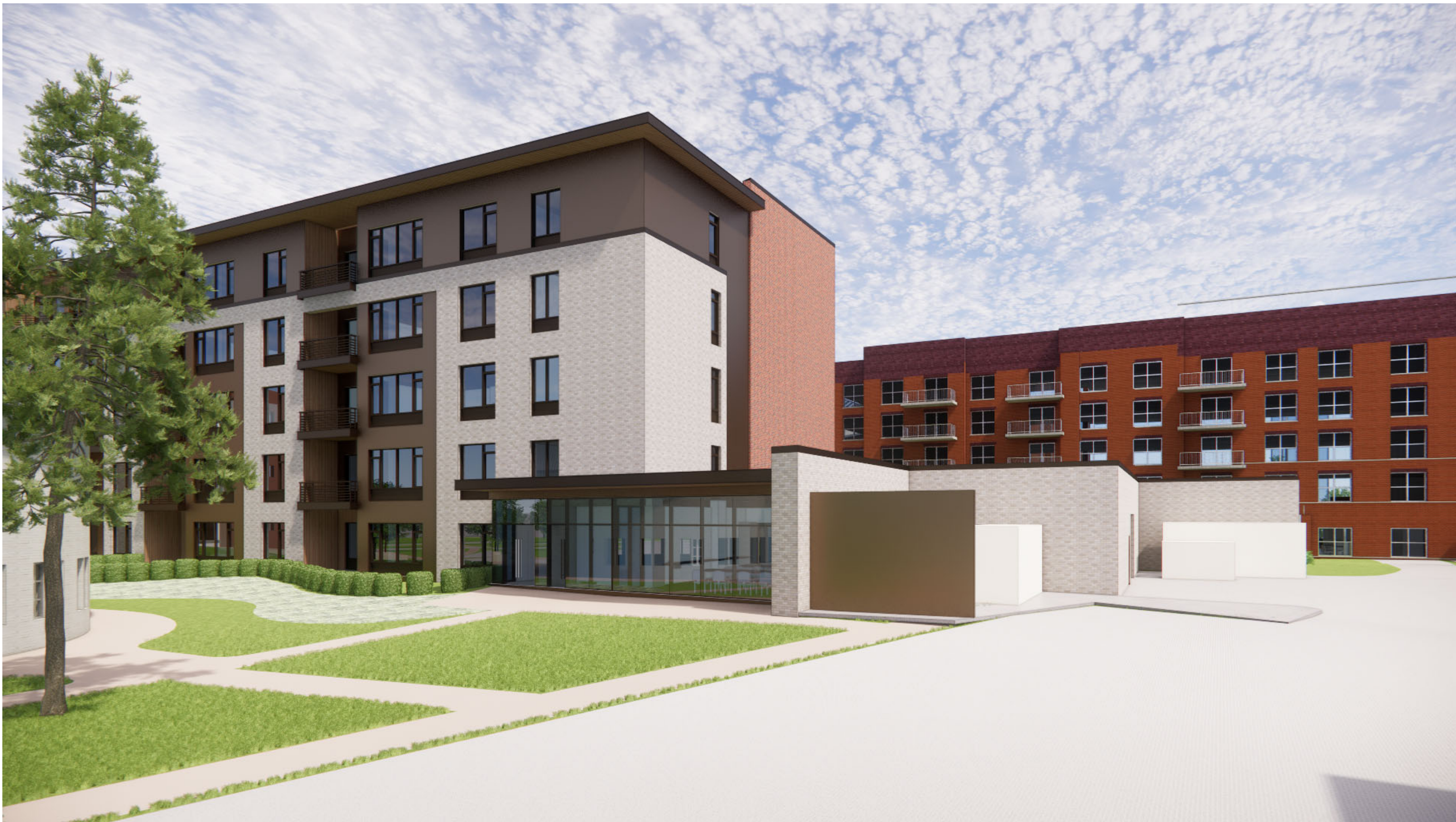
11. NORTH WEST VIEW
